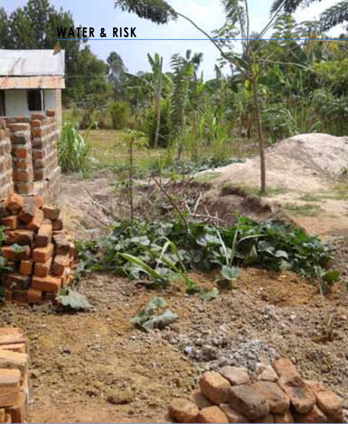
Figure 3: Brick production and wholes in soil Source: Sophie-Bo Heinkel
